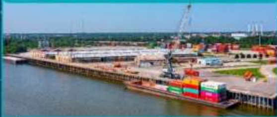
RICHMOND MARINE TERMINAL
